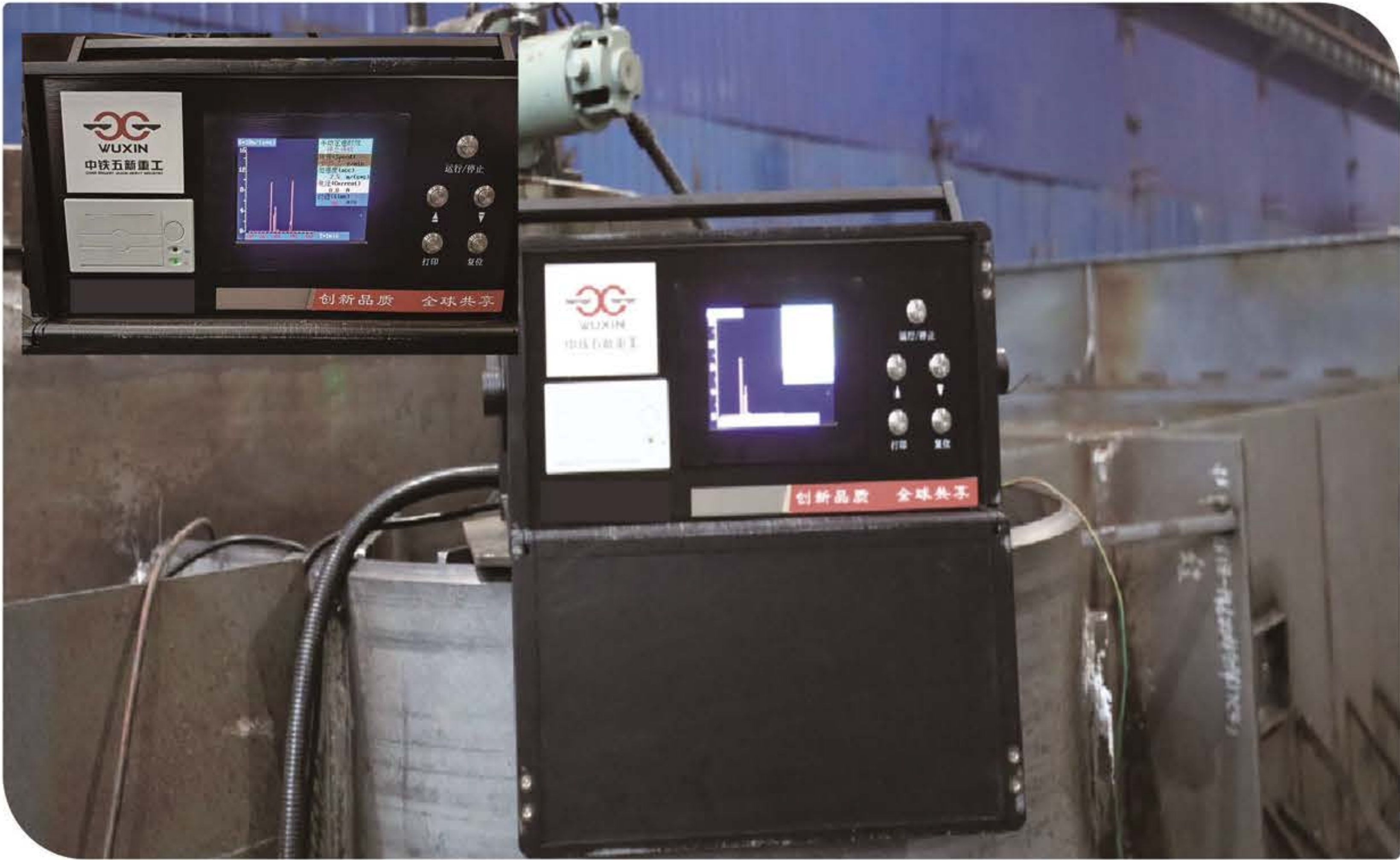
■ Welding Stress Relief
